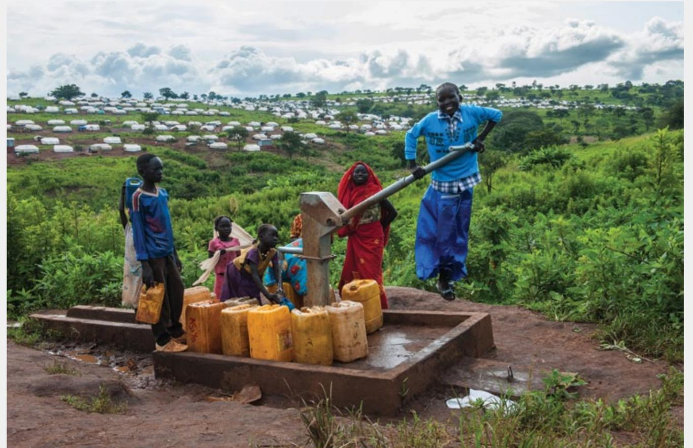
Boreholes equipped with hand pumps provide a source of drinking water.
