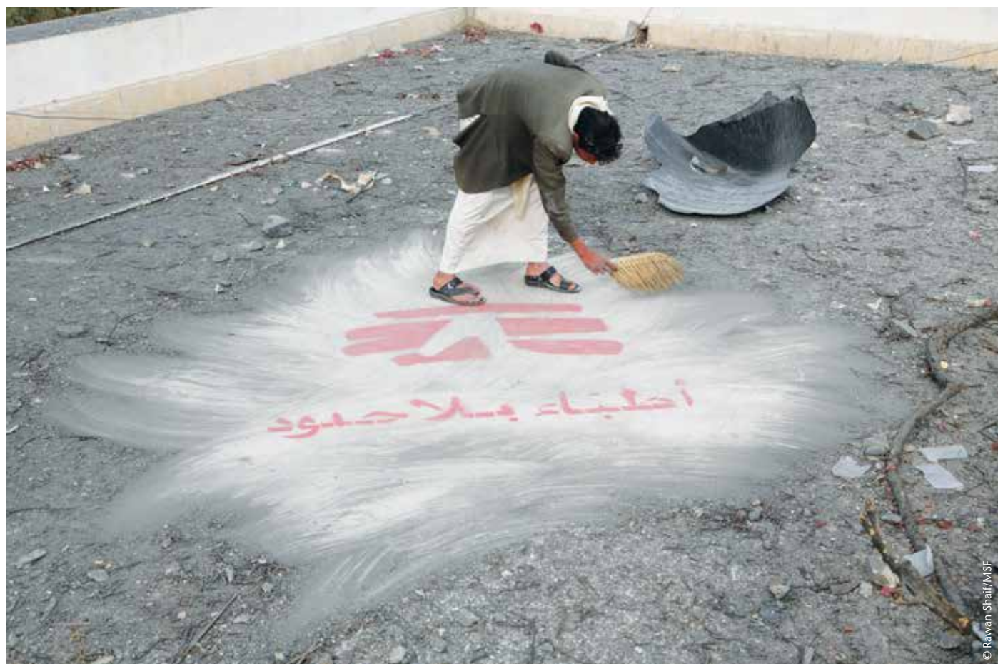
A man clears debris revealing the Médecins Sans Frontières (MSF) logo on the roof of an MSF-supported hospital in Haydan, Yemen after it was completely destroyed by an airstrike.
